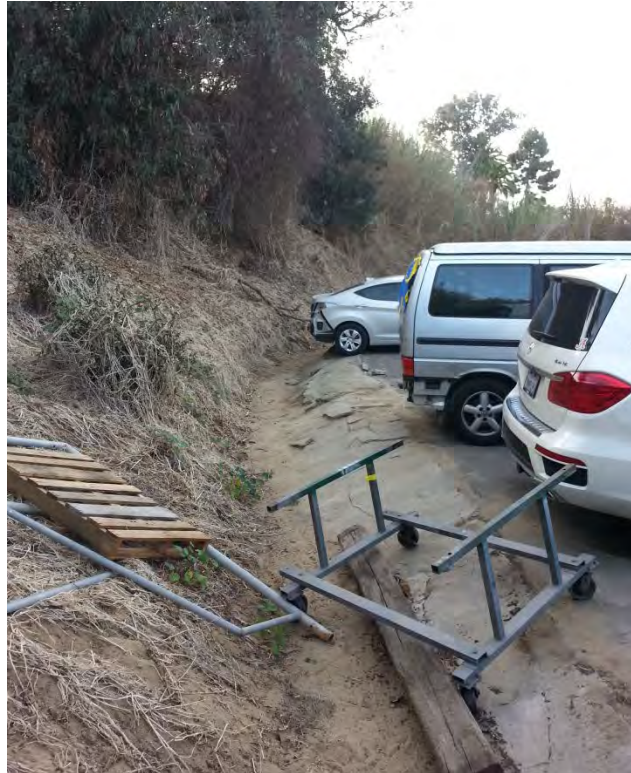
Figure 5. Partially concrete-lined drainage channel at edge of parking lot. View looking south from central-east part of project area.
