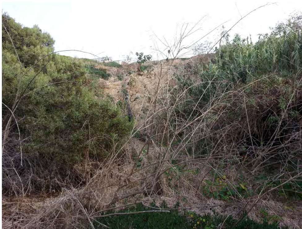
Figure 4. Head of drainage at northwest corner of property. View looking north. Note flexible black pipe in center of photo terminating partway down the slope.
